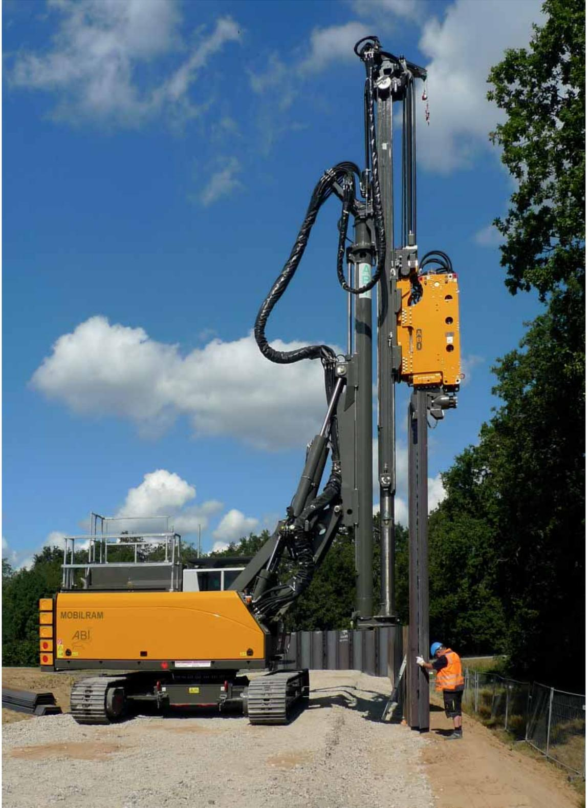
A classical application for the ABI MOBILRAM-System with vibrator: The installation of a sheet pile wall.
