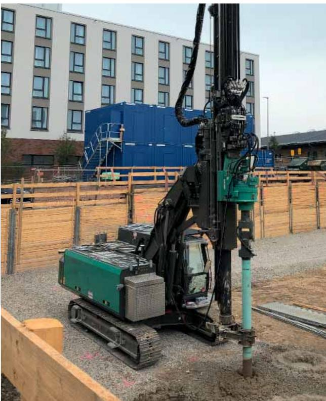
Increasing the load bearing capacity of the soil with mixed piles. Existing soil is mixed with aggregates while drilling and extracting.
