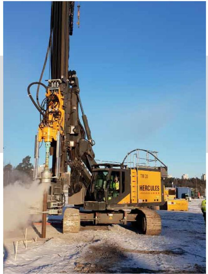
In hard, rocky soils down-the-hole hammers (DTH) are used for drilling.
